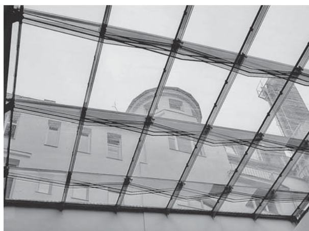
Fig. 3. Courtyard roof covering in Munich, Germany (photo by T. Serafinavičius)
