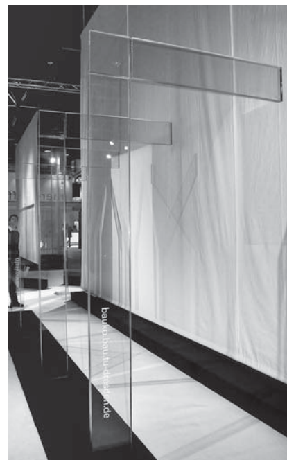
Fig. 7. Laminated structural glass column and beam with adhesive connection in Glastech-2010 (photo by T. Serafinavičius)
