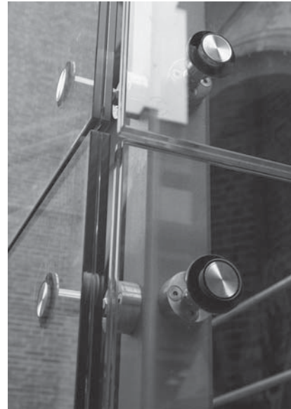
Fig. 6. Point-fix connection to tempered and laminated structural glass (photo by T. Serafinavičius)
