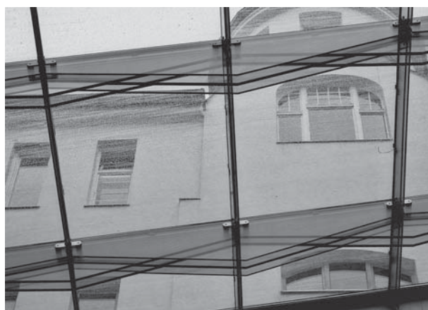
Fig. 4. Glass beams in roof construction, Munich (photo by T. Serafinavičius)
