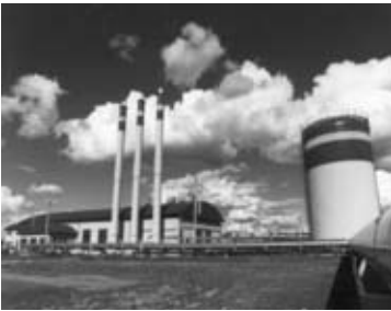
Fig. 7. Geothermal Power Plant
