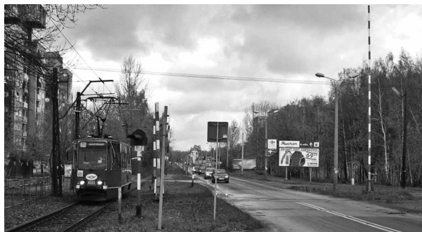
Fig. 2. Railway crossing on the tram route in Sosnowiec
