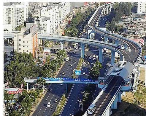
Elevated fully separated, RoW A busway, Xiamen
